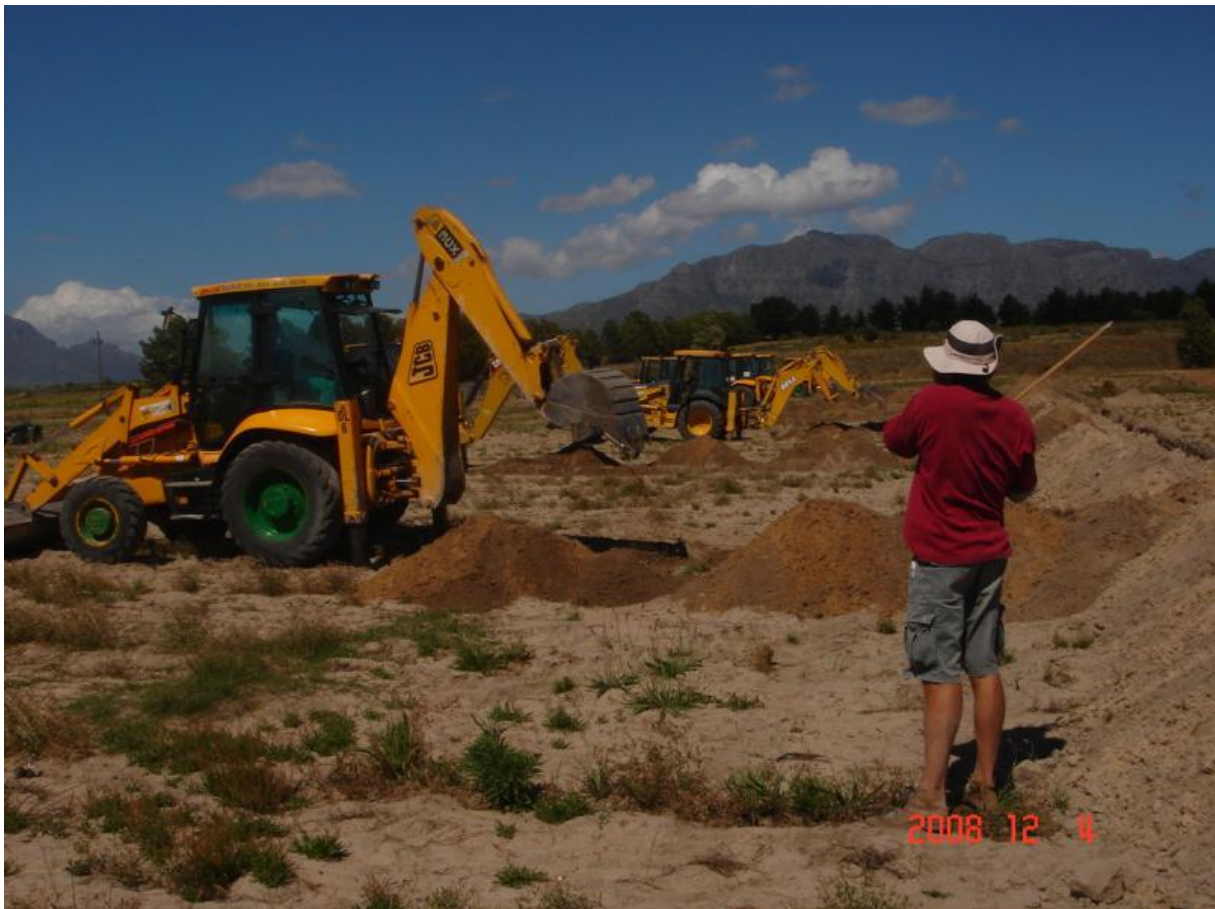
Figure 1: The degraded land prior to the project and the establishment of pastures using high density grazing. The machinery is being used to establish irrigation infrastructure.
